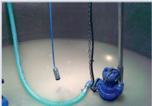
Pump on sliding pipe / level measurement pressure sensor
