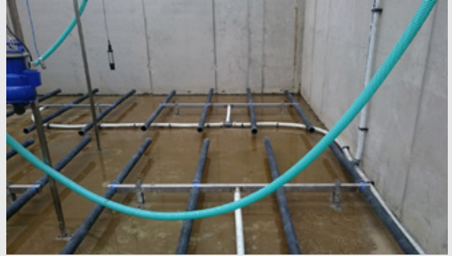
Aeration grid with membrane tube aerators in SBR
