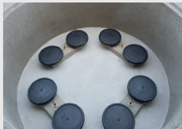
Aeration system with disc diffusers in the SBR reactor
