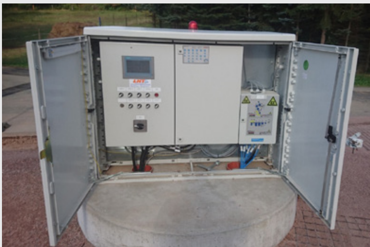
Outdoor column with control cabinet mounted on the technical shaft
